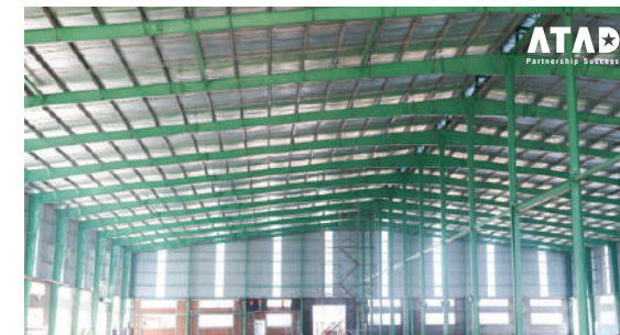
MANH PHUONG ELECTRICITY FACTORY PROJECT
