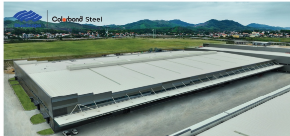
Project: THANH CONG - VIET HUNG AUTOMOBILE FACTORY
