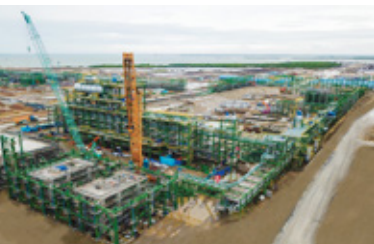
Long Son Petrochemical Complex
