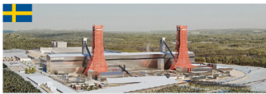
GREEN STEEL PLANT - H2GS - SWEDEN Scale: 5,000 MT
