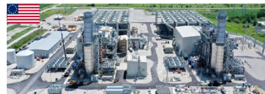
JACKSON GENERATION POWER PLANT - USA Scale: 3,760 MT
